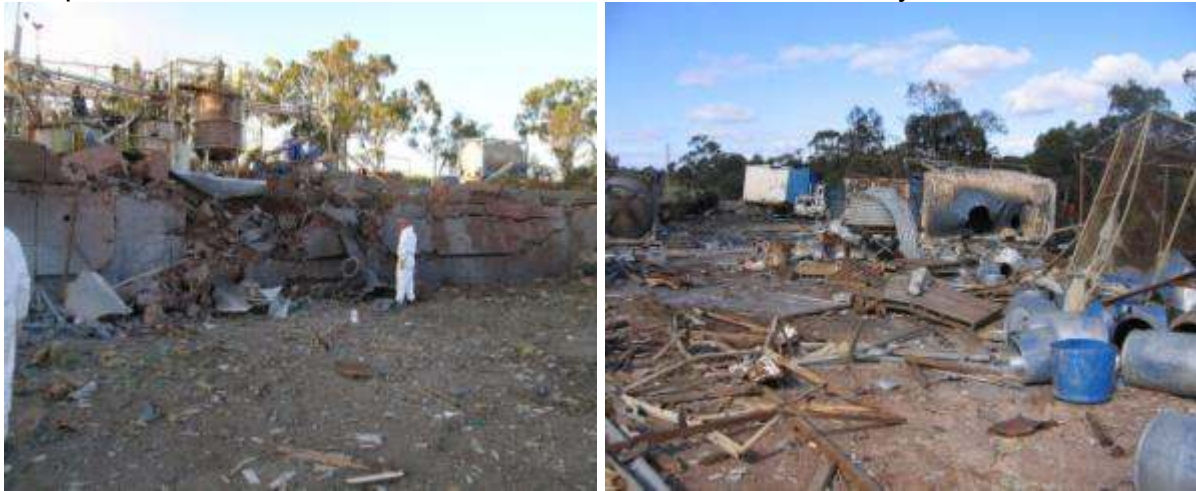
(L) the blast site with the damaged retainer wall, and (R) debris around the site, including the burnt shipping storage containers that stored TNT.
